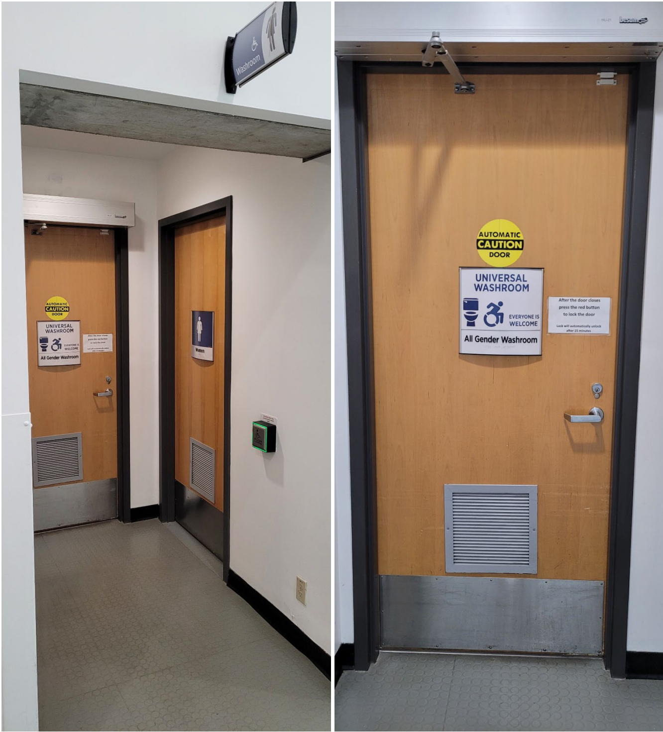
These are the washroom doors
